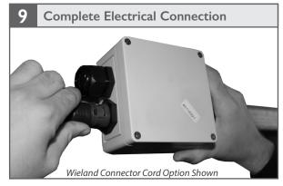
• Connect power cord from fixture to power supply.
